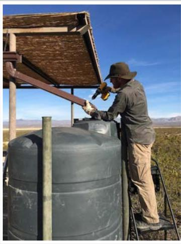
December 15, we completed installation of a 500-gallon rainwater storage tank. Using new gutters, this tank collects water that falls on one small section of the roof of the storage building near the parking lot. Even this small catchment area of 112ft<sup>2</sup> can result in 70 gallons of water
